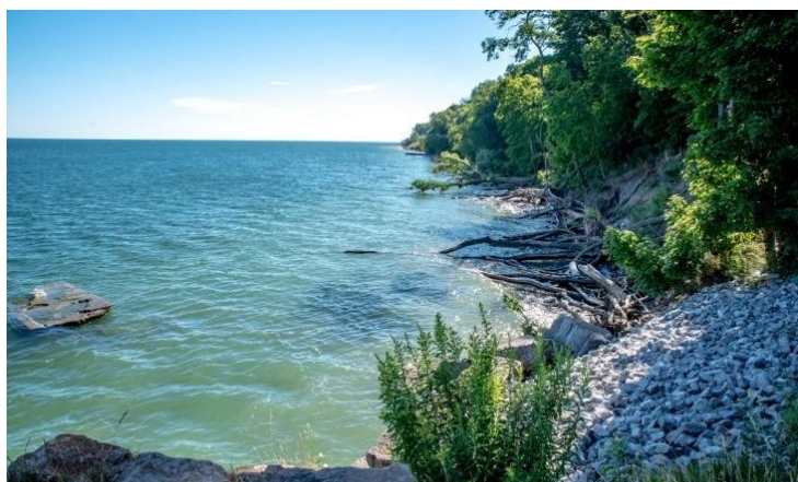
Figure 4. Erosion along the Lake Ontario shoreline at Old Fort Niagara (U.S. Army Corps of Engineers)
