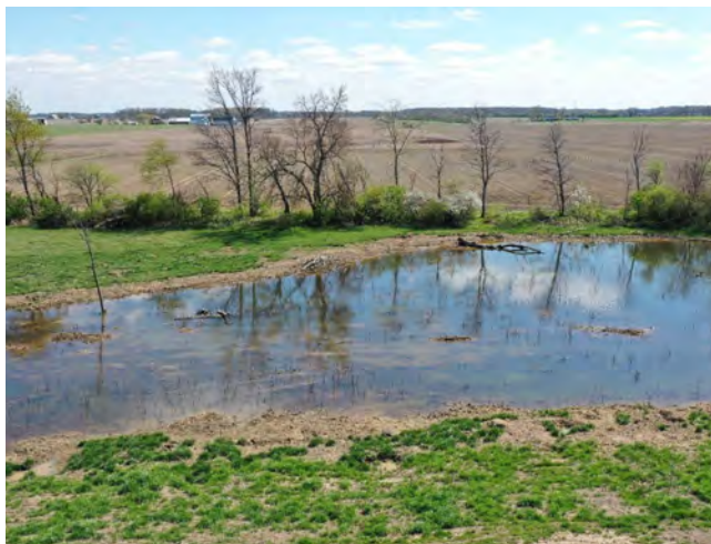
The Fruth Wetland Nature Preserve – an 18-acre wetland restoration project in Seneca County, Ohio – filters agricultural runoff from surrounding farm fields and reduces sediment and nutrient loads to western Lake Erie. Source: ODNR.
