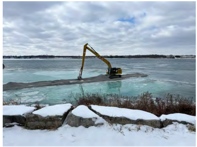
Capping of contaminated sediment at St. Clair River. Credit: CWA.
