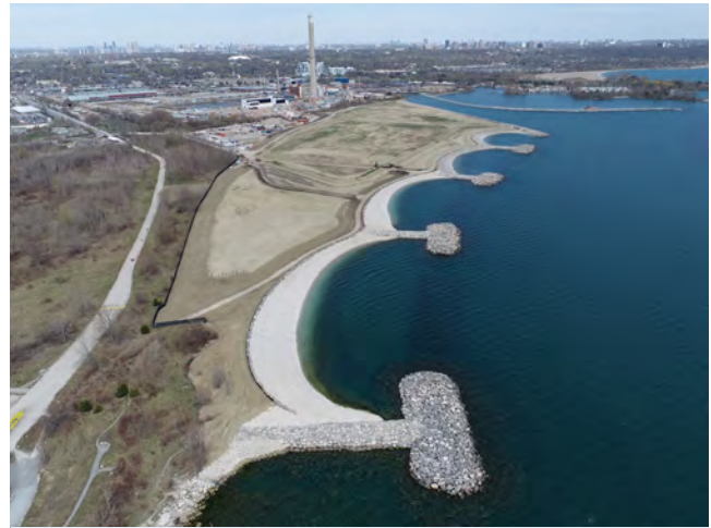
Erosion control structure along Ashbridges Bay Landform. Credit: Toronto and Region Conservation Authority.
