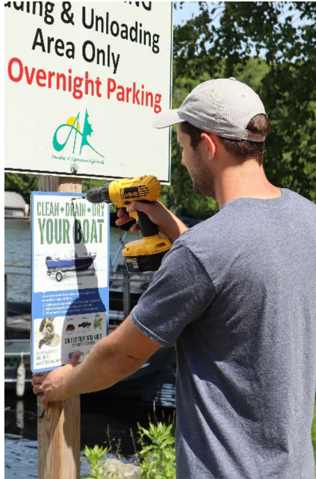
ISAP Volunteers install "Clean, Drain, Dry" signs. Source: OFAH.
