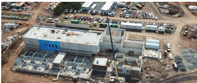
The Tertiary Treatment Building undergoing upgrades. Source: City of Hamilton.
