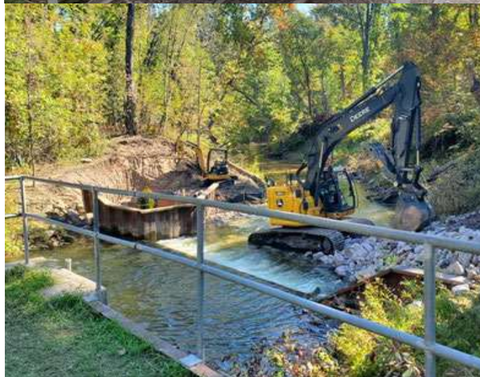
Top: A Sea Lamprey Trap. Below: The construction activity taking place to prepare the site for Sea Lamprey trap installation. Source: USACE.
