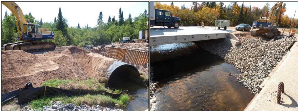
Top photo: Falls River culvert on Golf Course Road, Baraga County, Michigan, before removal. Bottom photo: Falls River Golf Course Road after culvert removal. Credit: E. Johnston, Keweenaw Bay Indian Community.
