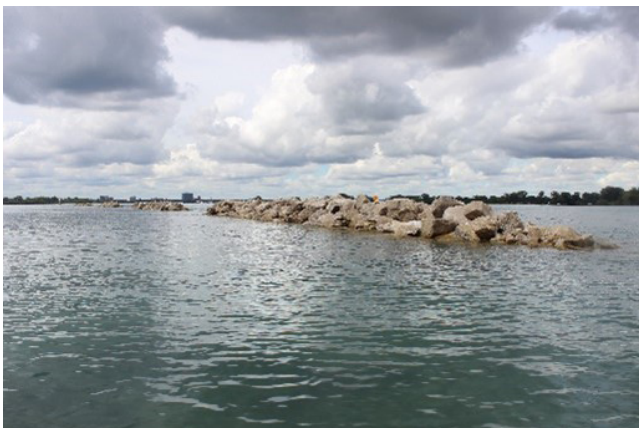
Four shoals created to protect Peche Island from erosion and create sheltered areas for fish and wildlife habitat. Credit: Jacqueline Serran, Essex Region Conservation Authority
