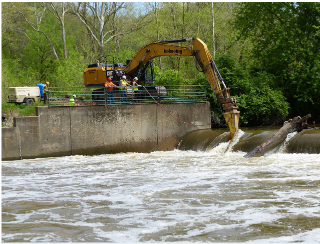
Crew begins removal of the Brecksville Dam structure. Credit: NPS
