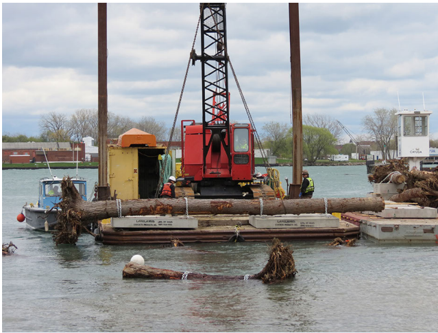
Log structures were installed at Spicer Creek Wildlife Management Area to deflect wave energy. Credit: NYSDEC
