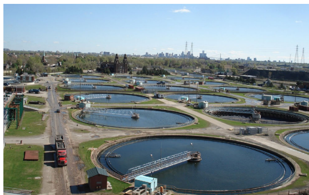
View of secondary clarifiers at the Great Lakes Water Authority's Water Resource Recovery Facility. Credit: Michigan EGLE
