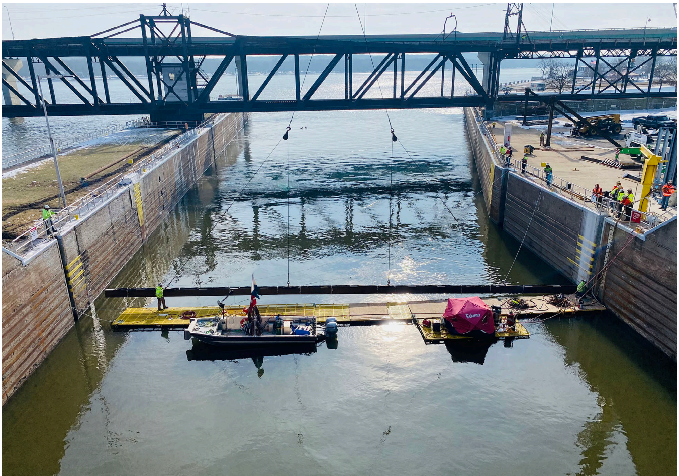
Installation of a multi-speaker soundbar at Lock 19 on the Mississippi River (Keokuk, Iowa), February 2021. This project is testing a prototype underwater acoustic deterrent system at a known invasive carp fish passage “pinch-point”. Credit: Marybeth Brey, USGS
