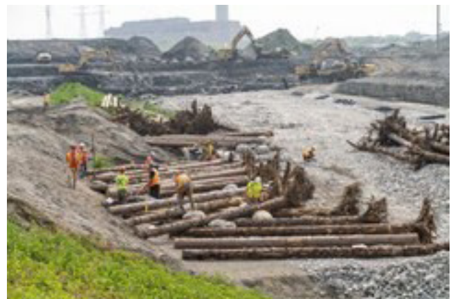
Tree logs being placed on sides of new river channel to create habitat for wildlife and shelter for fish, Don River Mouth Revitalization, Toronto and Region Area of Concern, Lake Ontario. Credit: Waterfront Toronto
