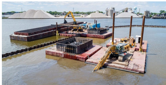
Remediation of contaminated sediment at a former manufactured gas plant site in the Fox River AOC. Source: JF Brennan
