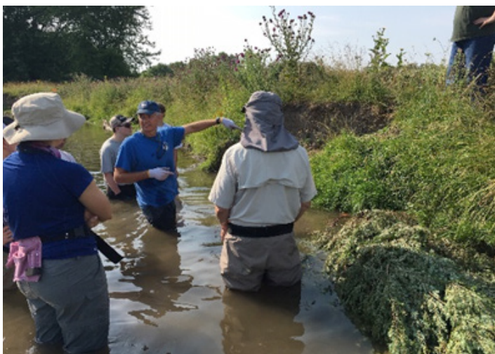
Photo of Bank stabilization using discarded Christmas trees & soil anchors. Source: NVCA.
