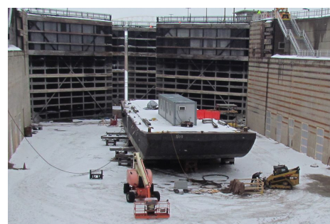
Réparations écluses de "Soo" (credit: USACE).
