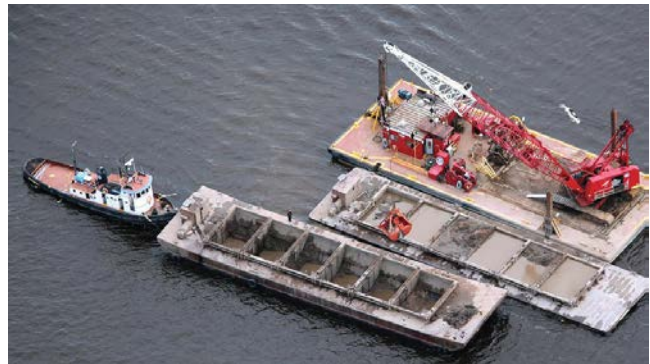
Dredge material sourced from the East Gate Basin was placed at the 40th Avenue Site in the Summer of 2017. Credit: Nelson French, previous AOC coordinator.
