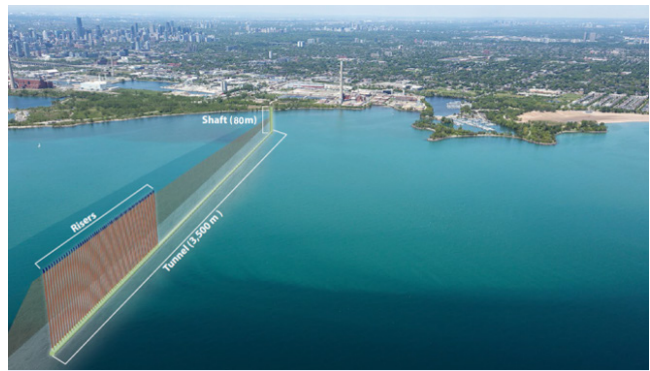
Construction of the new outfall at Ashbridges Bay wastewater treatment plant. Credit: Hatch with CH2M and Baird.
