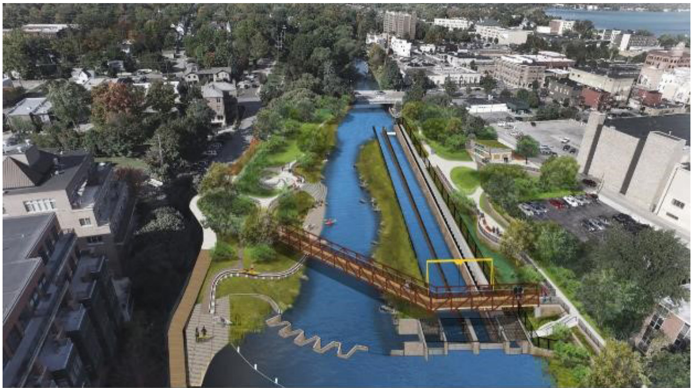
Birds-eye rendering of the 65 percent engineering design of FishPass featuring an adaptive fish-sorting channel (right) and nature-like bypass channel (left). Fish passage and flow is ultimately regulated at FishPass by an arced-labyrinth weir (lower left) and dual hydraulic gate system (lower right). Credit: USACE, City of Traverse City, GLFC and AECOM.
