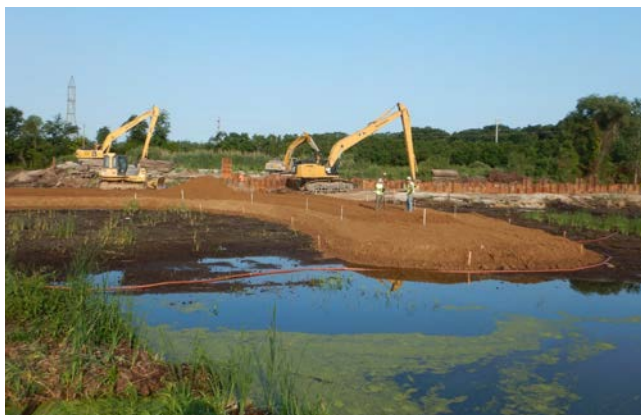
Contractors complete sediment cleanup work and begin prepping the wetland. Credit: USEPA.
