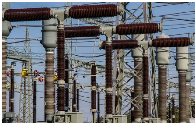
PCBs have been used to make coolants and lubricants for certain kinds of electrical equipment, such as transformers and capacitors. Credit: Th G, Pixabay.
