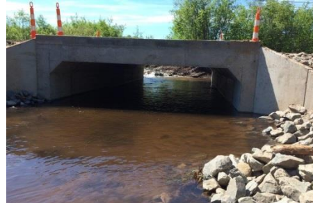
The culvert (above, before) on Menge Creek was removed to restore natural flow (below, after). Credits: Keweenaw Bay Indian Community.
