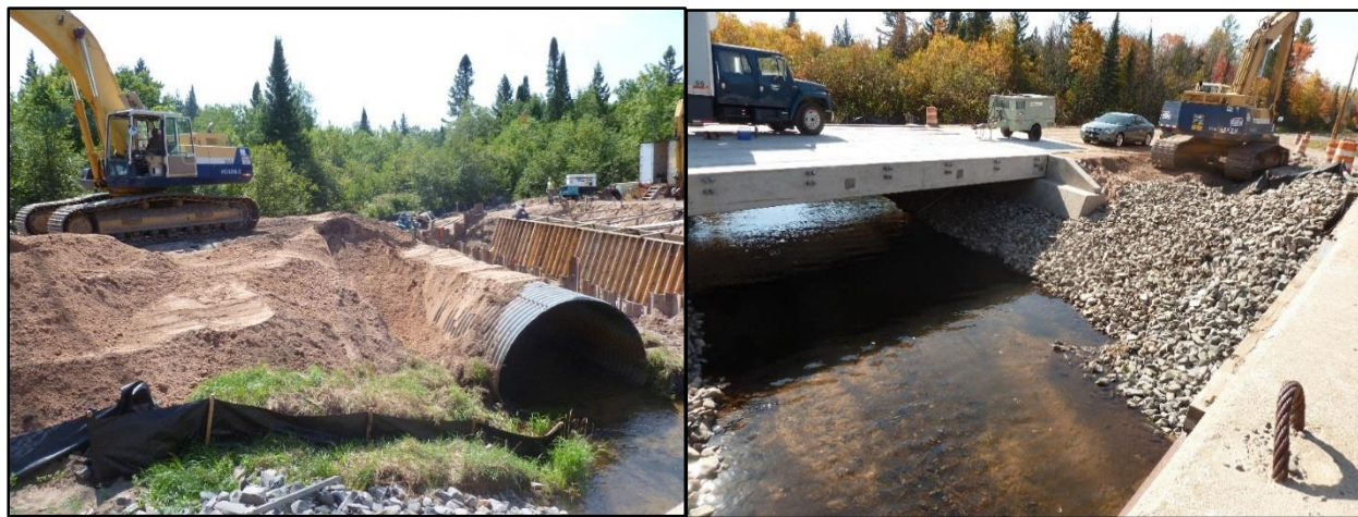
Left: Falls River culvert on Golf Course Road, Baraga County, Michigan, before removal. Right: Falls River Golf Course Road after culvert removal. Credit: E. Johnston, Keweenaw Bay Indian Community.
