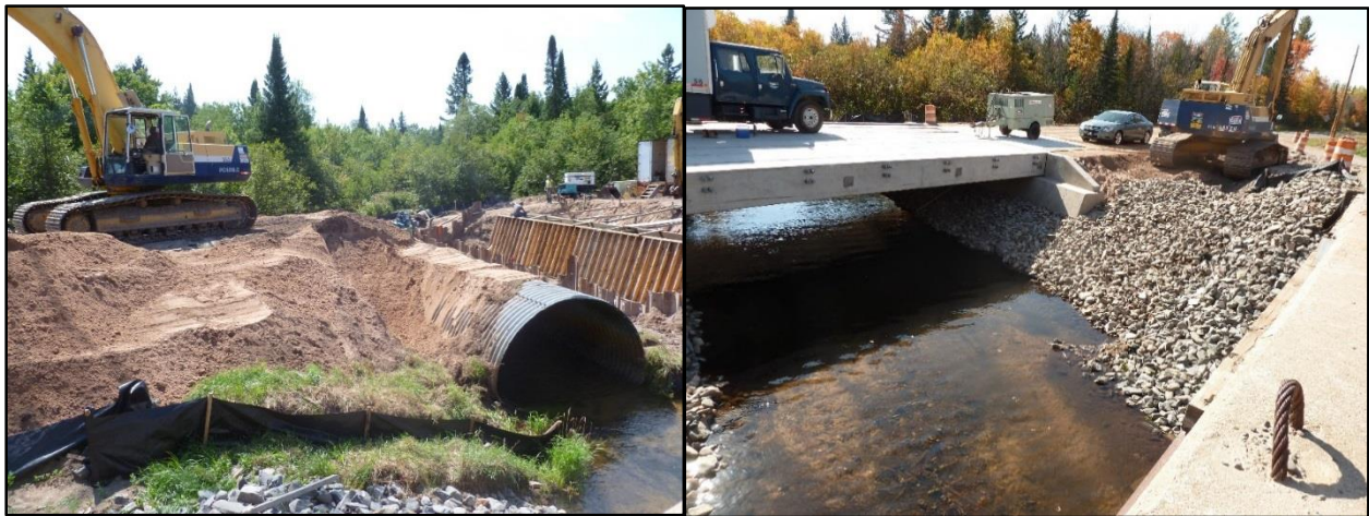
Left: Falls River culvert on Golf Course Road, Baraga County, Michigan, before removal. Right: Falls River Golf Course Road after culvert removal. Credit: E. Johnston, Keweenaw Bay Indian Community.
